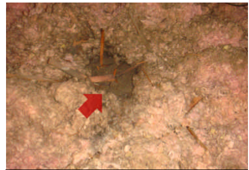
Shower stall ceiling vent screen in attic.
