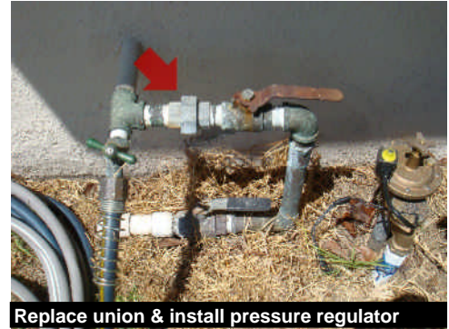
Replace union & install pressure regulator
