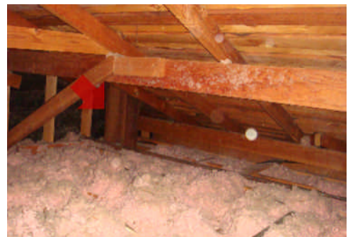
View of the kitchen ceiling exhaust duct.
